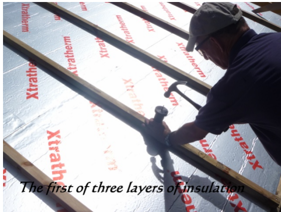
Above - roof insulation
