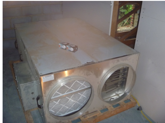
Heat Recycling Ventilation plant
