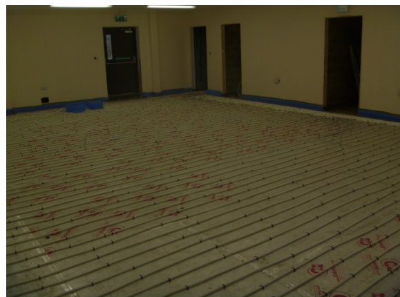
Underfloor heating installation
