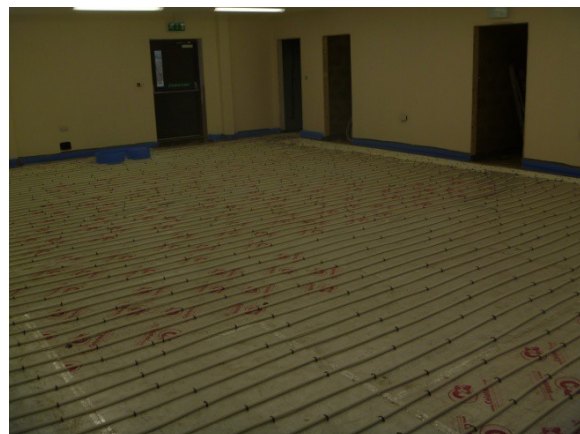
Underfloor heating installation
