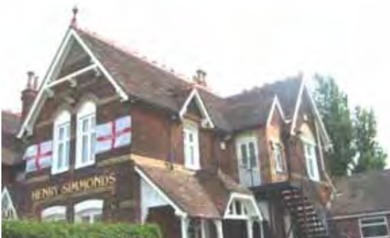
The commercial centre continues north of the railway line into Wrotham Road. The Henry Simmonds public house is a local landmark due to its scale, prominent gables, decorative ridge tiles and finials, half timbering and tall chimneys.
